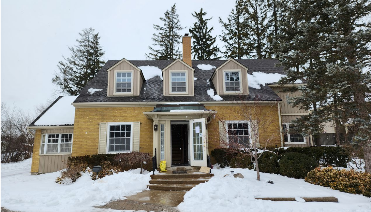
(Figure 2: Front façade of the existing building)
